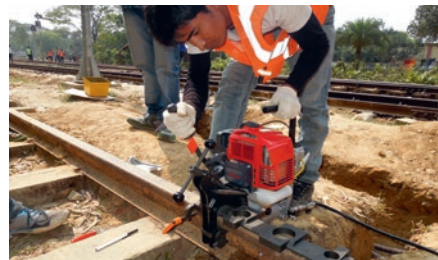
Drilling of the hole
